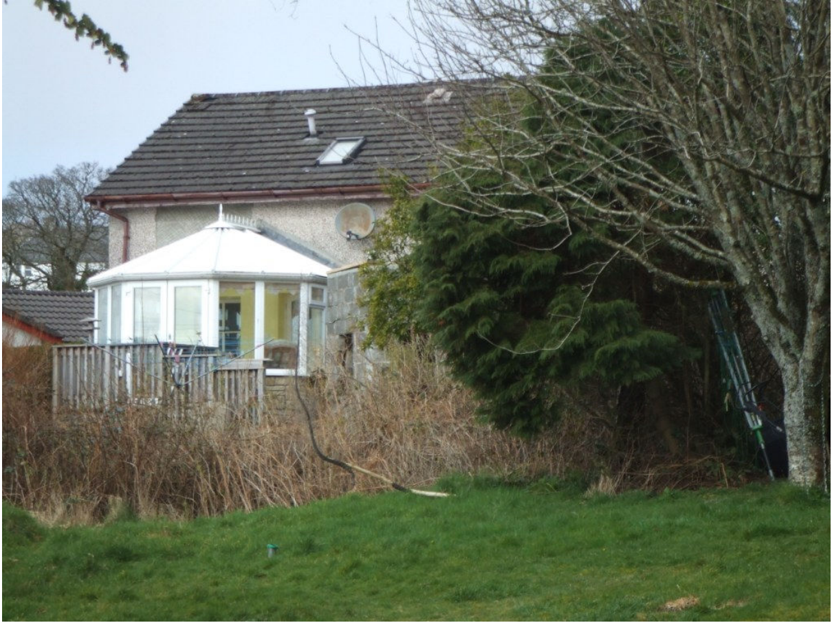
View from Trewince of conservatory during construction
